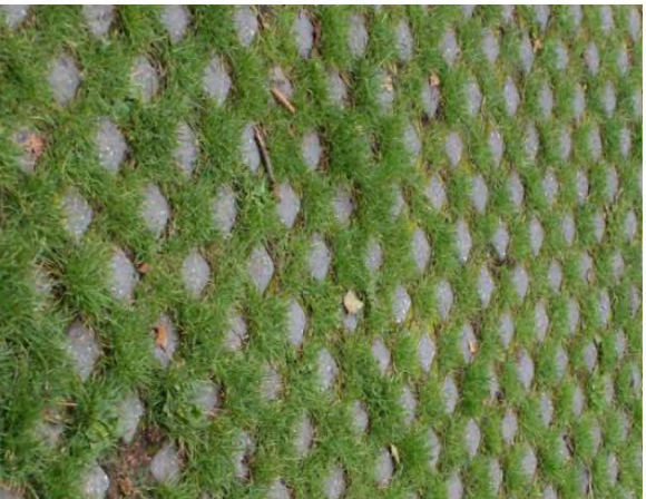
Graskeien halfverharding tpv parkeren
